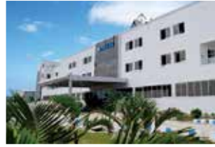
Rudrapur Plant (Green Building)
